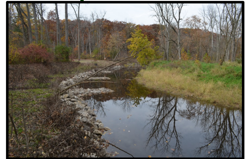
Ottawa River has erosion control structures
