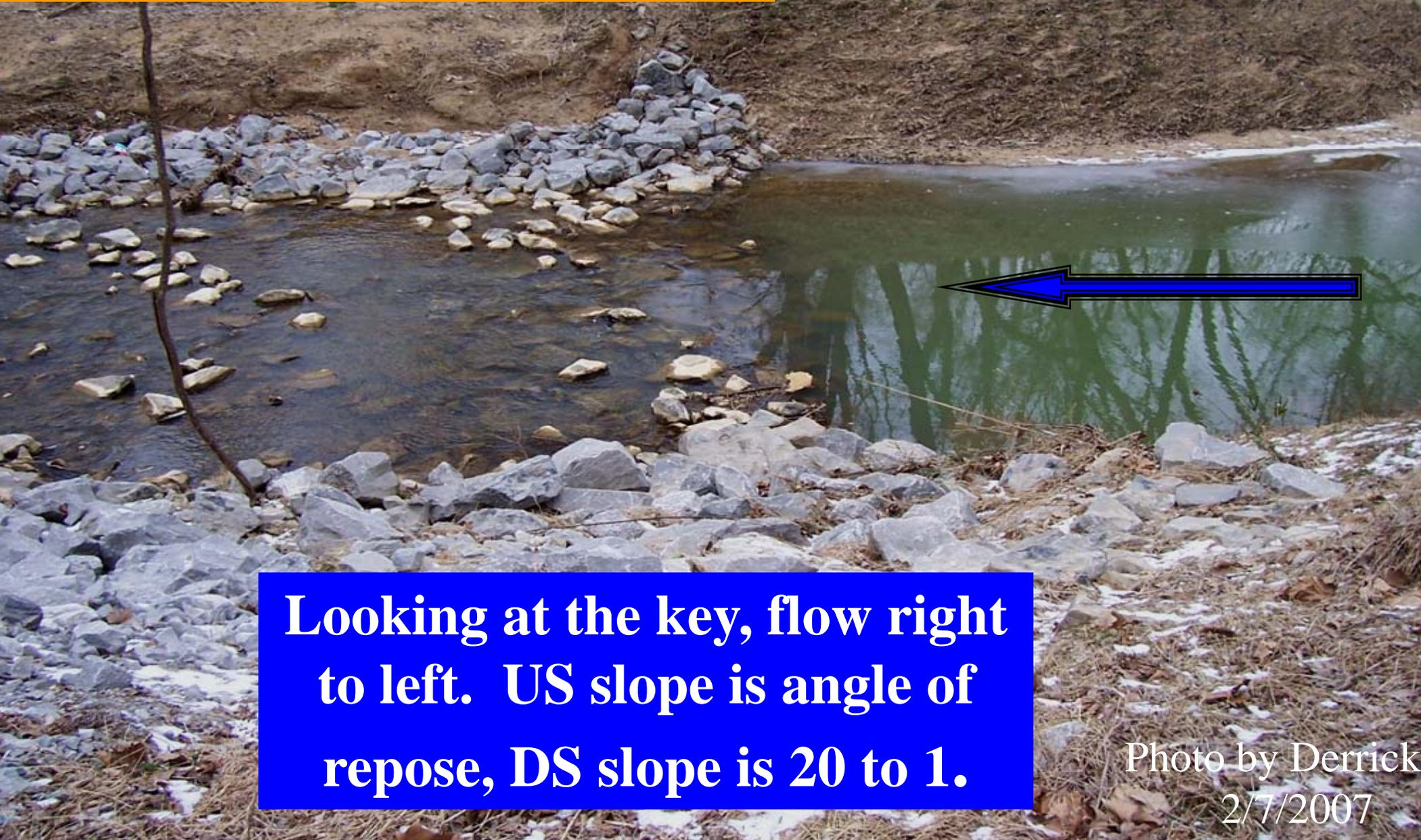
**Looking at the key, flow right to left. US slope is angle of repose, DS slope is 20 to 1.**
